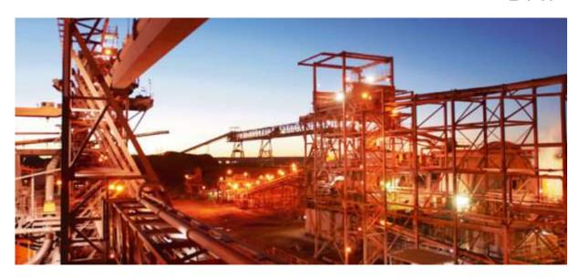
Smelter campaign maintenance- shutdown and repairs to the smelter including rebuilding key elements of the smelter flash furnace; demolishing and building a new electric slag furnace; and removing and replacing the five-story high electro static precipitator.
